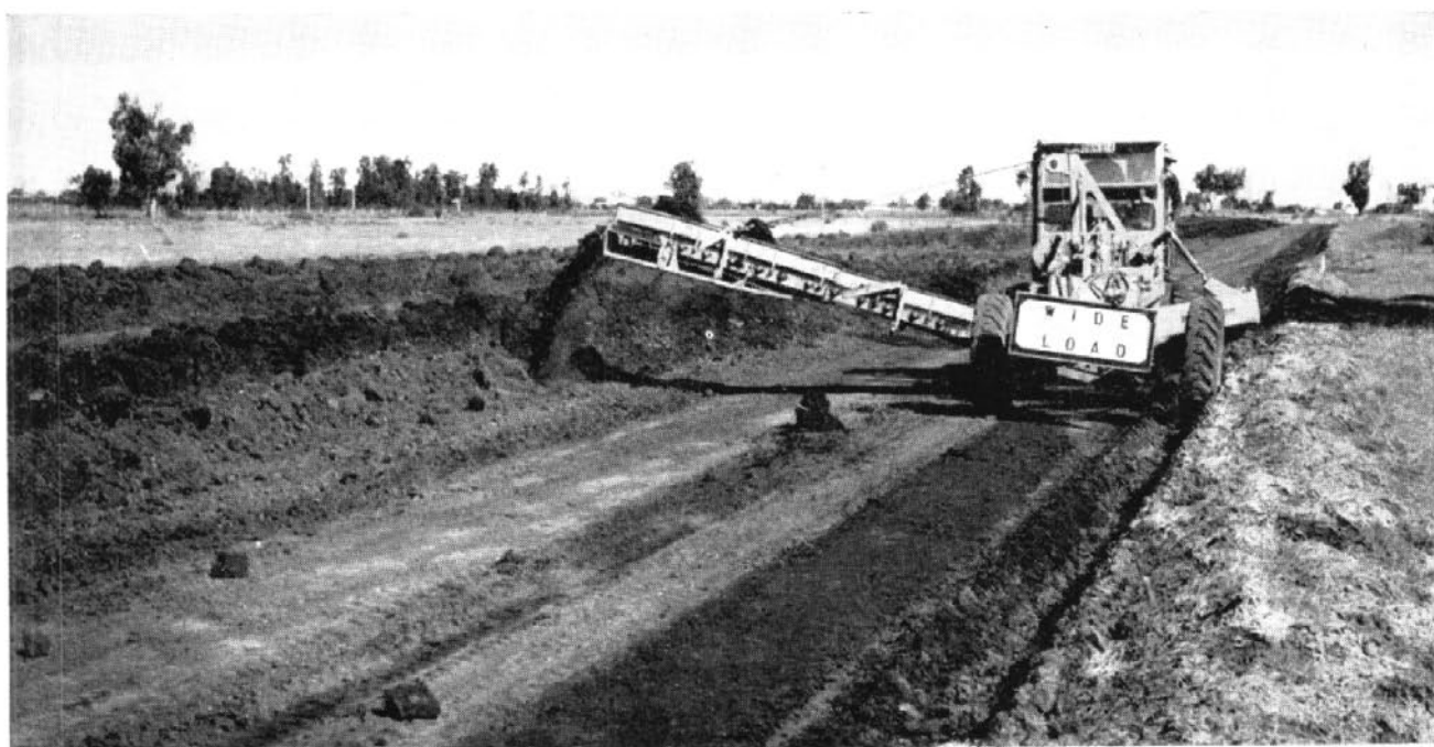
An elevating grader at work on the Castlereagh Highway north of Coonamble.
