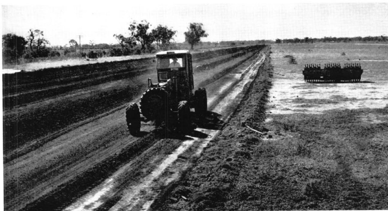
Road formation approaching completion on the Castlereagh Highway north of Coonamble.
