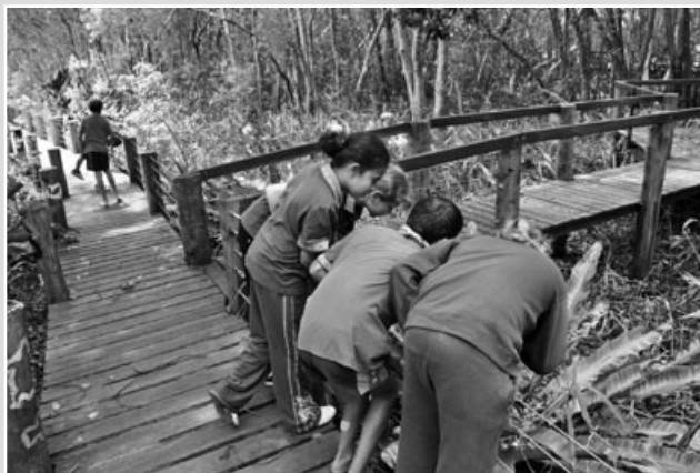
Cabbage Tree Island wetland boardwalk
