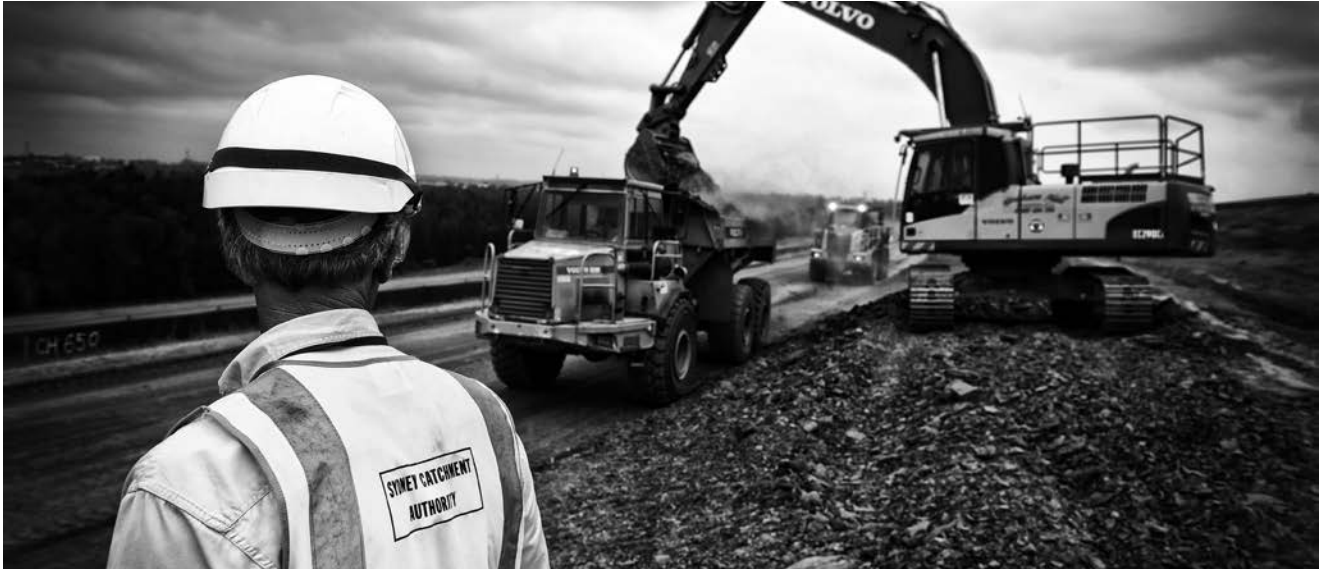
Major dam wall improvements were carried out at Prospect Reservoir
